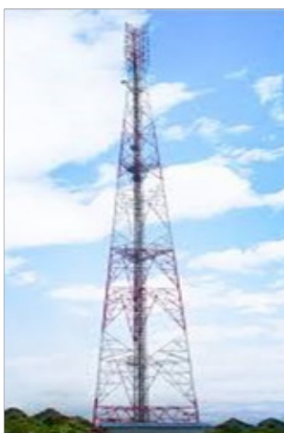
Menara kekisi berkaki tiga (three-legged lattice tower)
